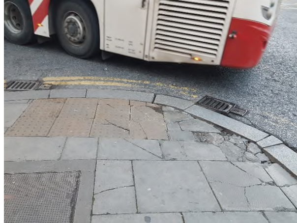
Damage to footpath at Store Street Junction
